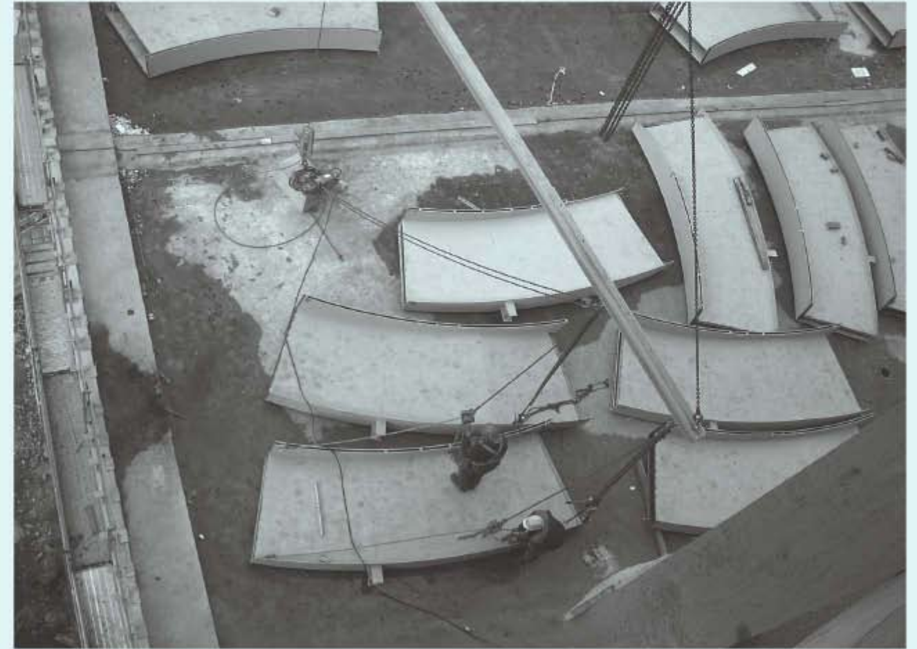
18 Montage der Innenrampe — Construction phase of inner ramp
