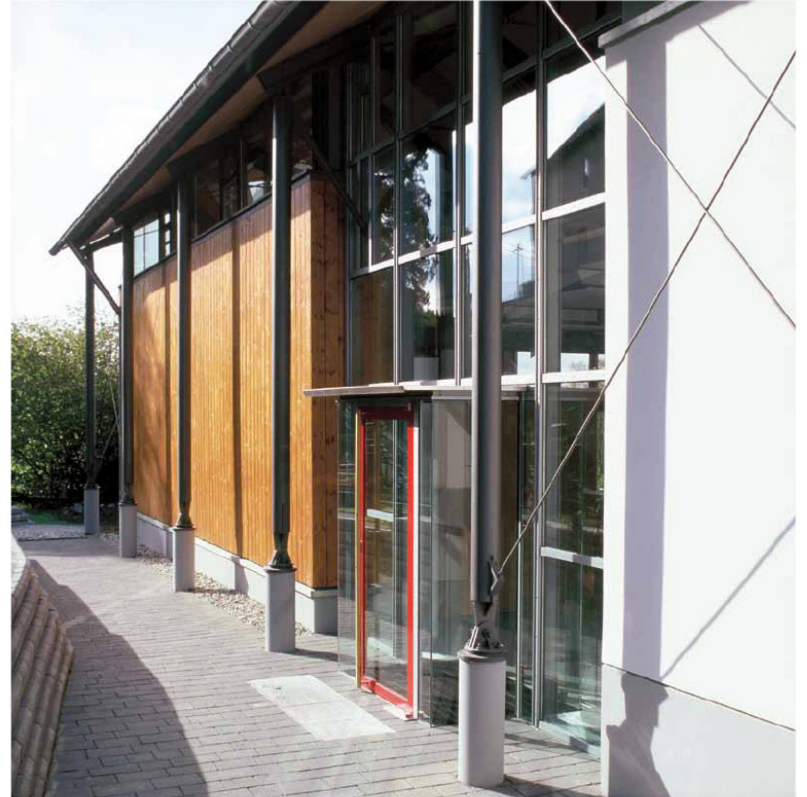
65 | 66 67 — Detailed views of the suspended girders
